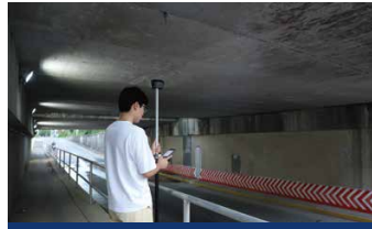
ROAD CONSTRUCTION SURVEYING
