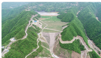
Tailings dam slope
